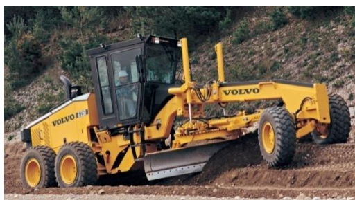
Figure 2. Ground leveling with grader.
